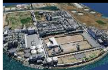
JACOBS AND PUB, SINGAPORE'S NATIONAL WATER AGENCY Tuas Water Reclamation Plant (TWRP)
