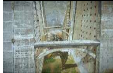
HDR Murray Dam Condition Assessment
