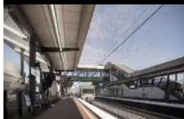
ACCIONA Safely Removing Dangerous Level Crossings through Digital Construction Victoria, Australia
